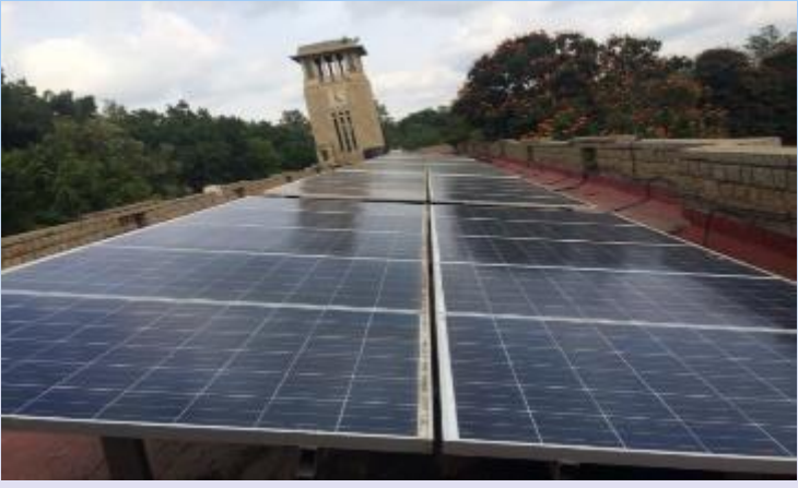
HAL – TERI CSR Initiative : 47 Public Schools installed with SRTPV systems 478 kWp
